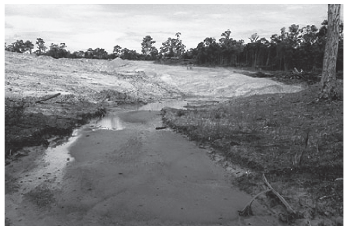
Eroded soil from land cleared for urban development has led to the accumulation of sediment in the gully at the foot of the slope. Source: EPA
